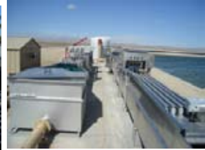
Commissioning 2 Reactors in Lancaster CA
