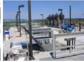
Commissioning in Watsonville CA
